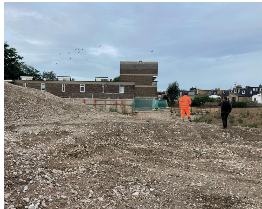
3 Current view looking towards Donnelly Court
