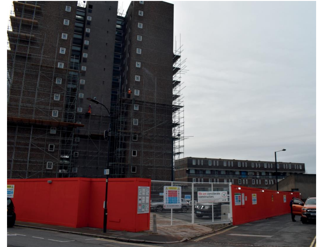
2 View looking down Williams Close during demolition
