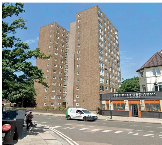
(A) View of the previous towers on site
